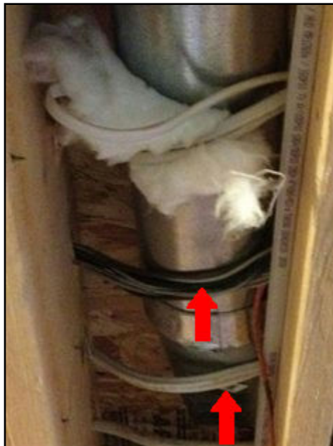
11. Too close to ducts, pipe, chimneys, etc.
