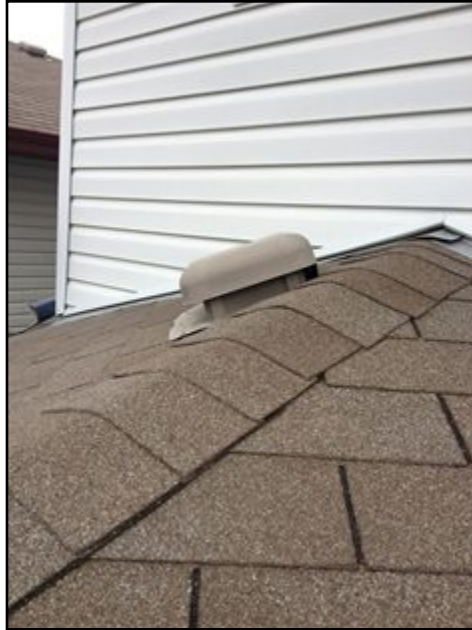
1. From roof edge
