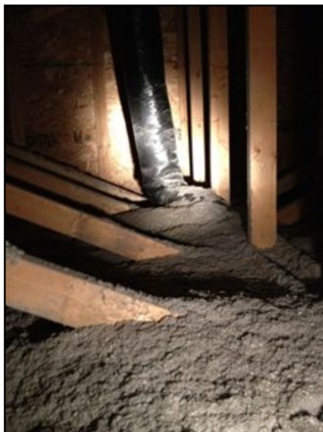
10. Inspected from access hatch
